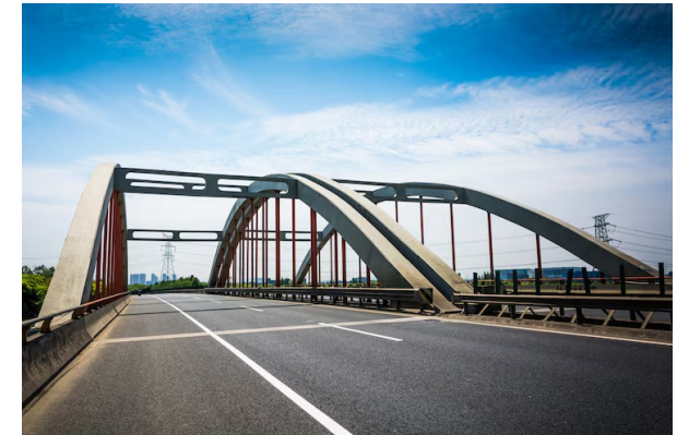
Bridges ,Roads & Infrastructure Development Works
