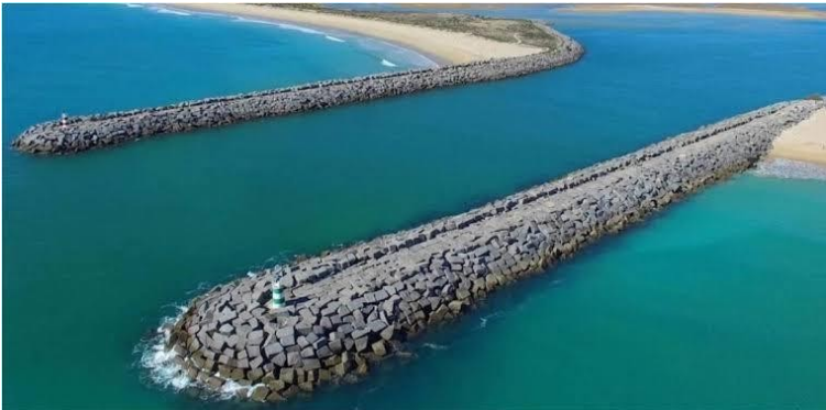
Shore Protection walls /Bait Arch/Break water
