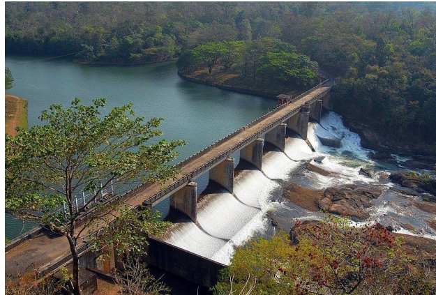
CHECK DAM & BRIDGES
